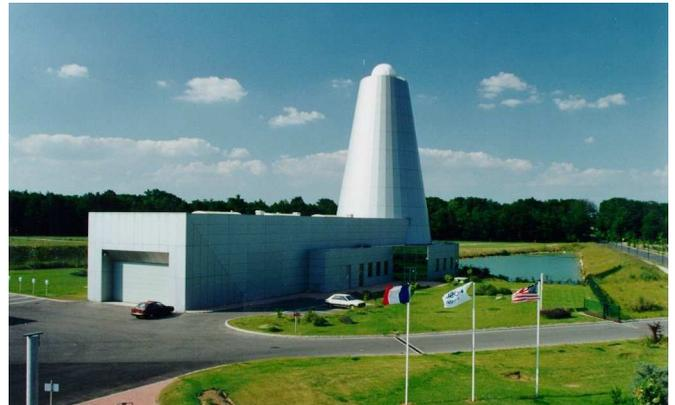
**The building** erection was achieved in April 1992. The shop is a 70-meter long building of about 1100m<sup>2</sup> total floor area with a 35-meter high tower at one end above the polishing machine. The shop also includes a grinding zone, a storage zone and a downloading zone. Offices are placed around the polishing zone.
